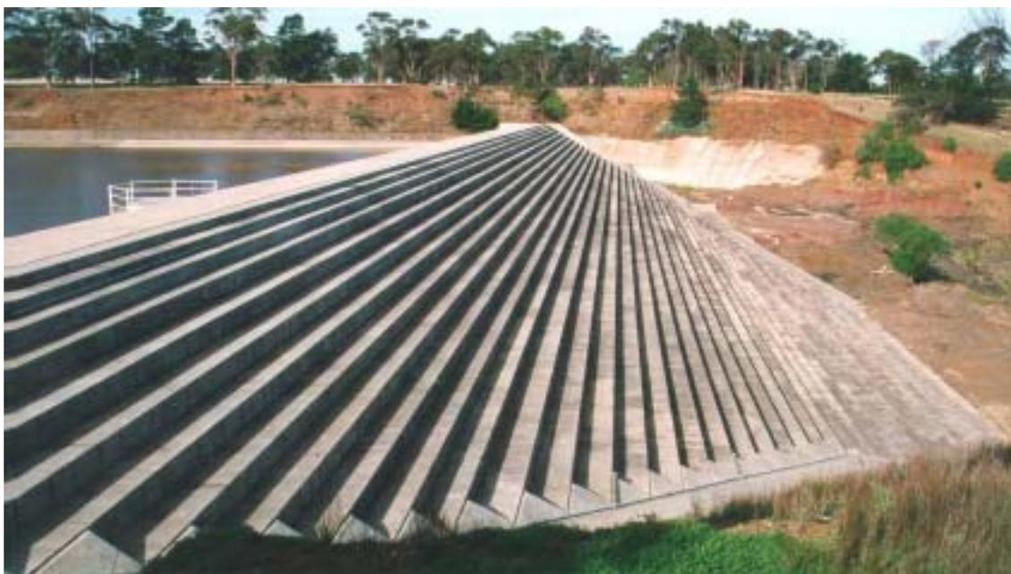
Figure 3 Melton dam stepped spillway on 30 January 2000—Completed in 1916, the Melton dam was equipped in 1994 with a secondary stepped spillway ( $Q_{\text{des}} = 2,800 \text{ m}^3 \text{ s}^{-1}$ ,  $h = 0.6 \text{ m}$ ).
