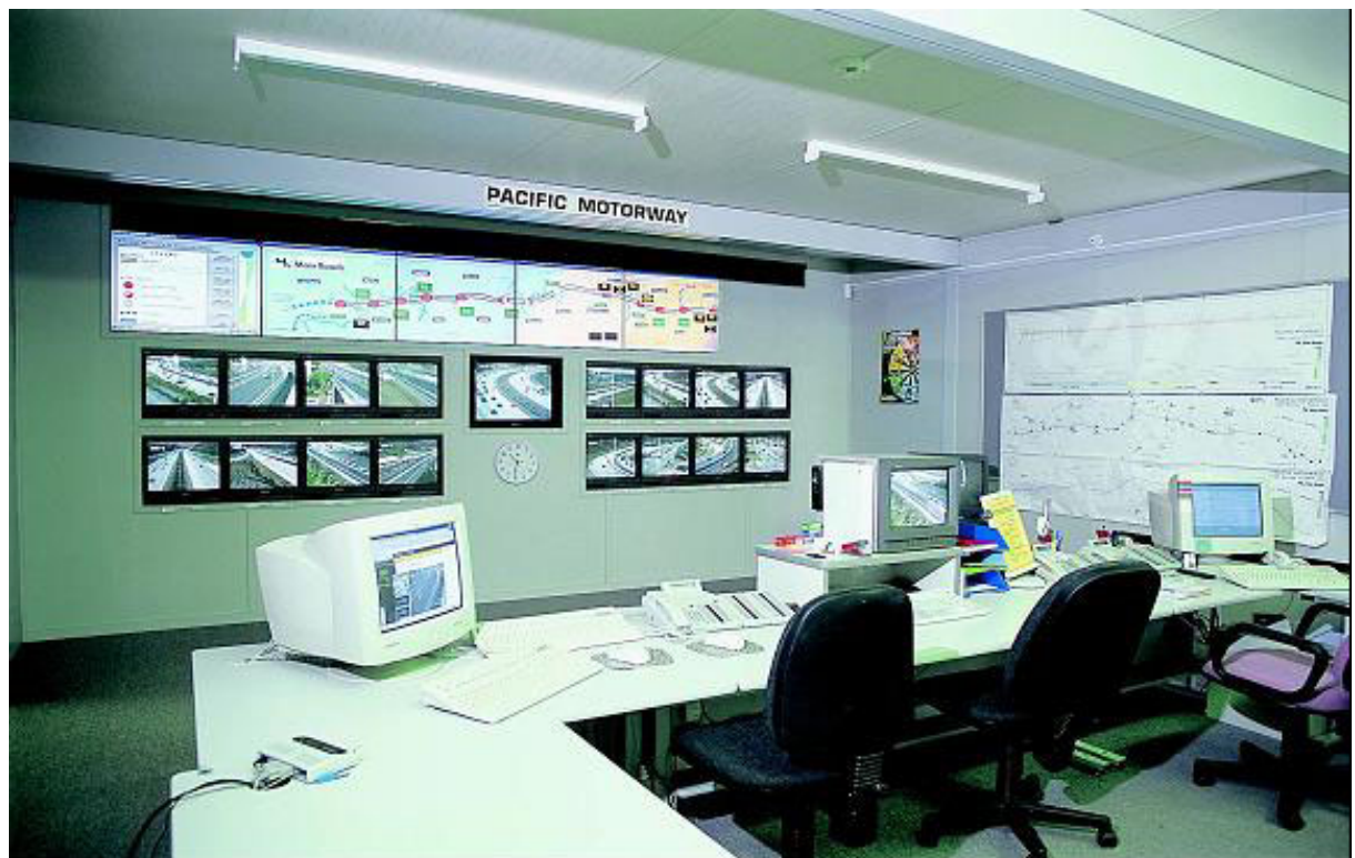
Figure 3 – Project Traffic Management Center
