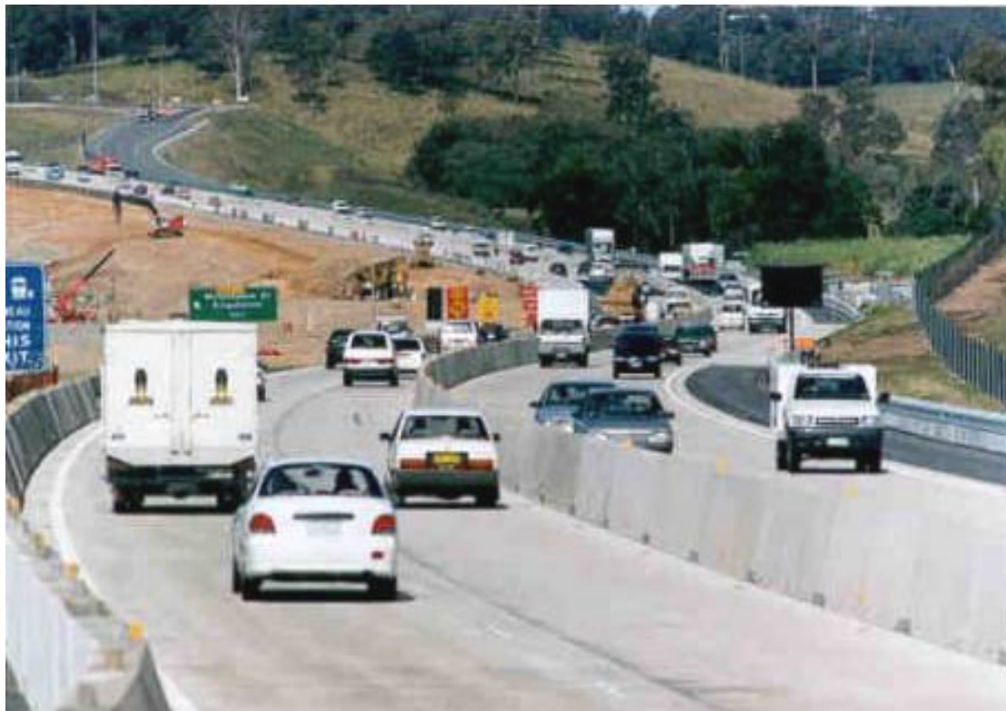
Figure 1 – Positive Separation by Concrete Barrier
